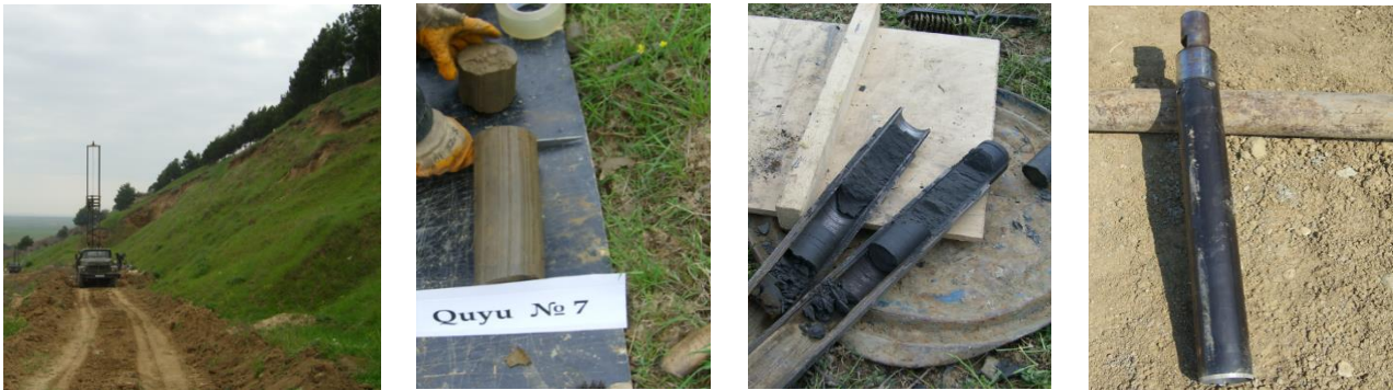
Figure 3. Episodes of geotechnical research on the slope
