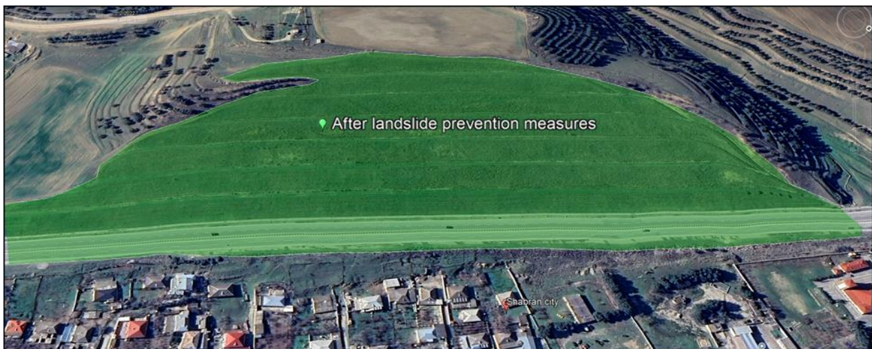
Figure 11. Image of the study area after landslide measures
